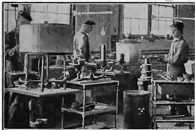
FIG. 20. FILLING THE SHELLS WITH ROSIN, AND SCREWING IN THE PLUGS
